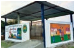
Centralized Material Collection Facility
