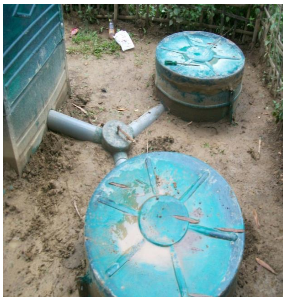
Sub Structure with FRP material
