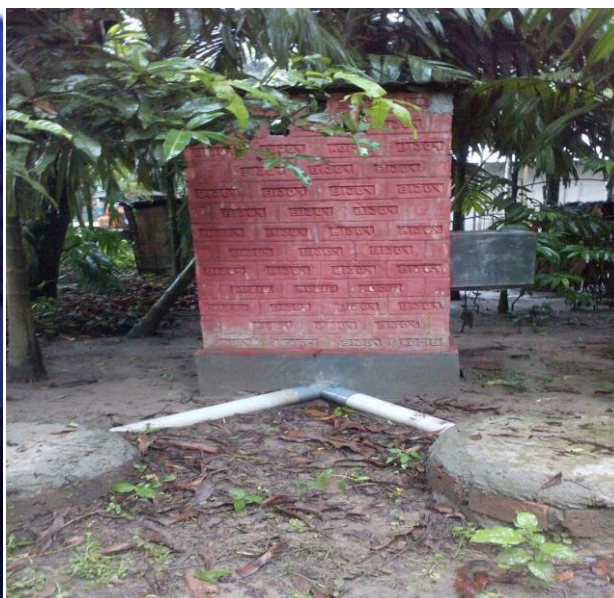
Toilet with PVC Changeover facility
