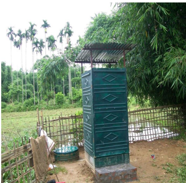
Super Structure with FRP material
